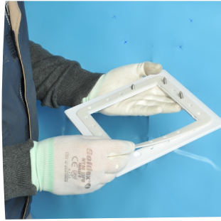
Place the seal over the flange
