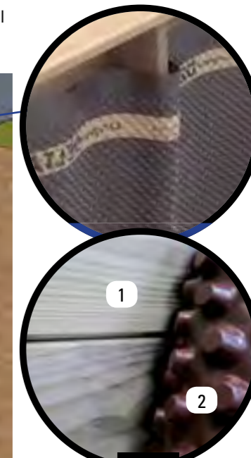
Fig. 6 1- Wood frame 2- Roll of alveolar protection and drainage of HDPE
