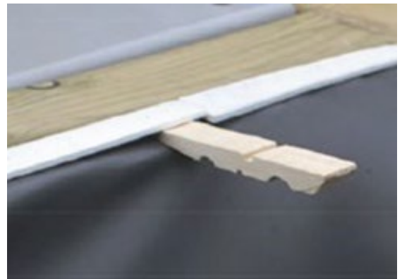
Figure 32 – Blocking the liner in position using half clothes pegs
