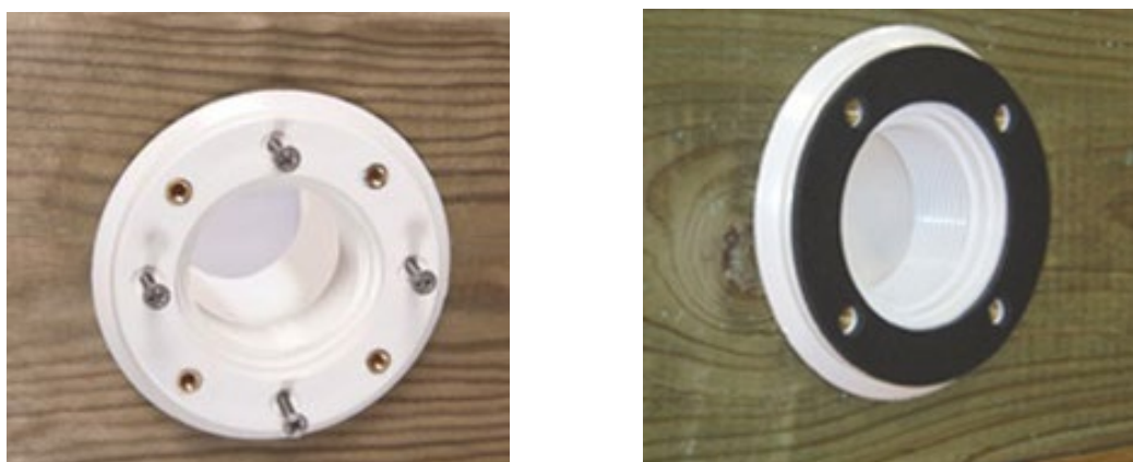
Figure 24 – Mounting the return fitting body and gasket
